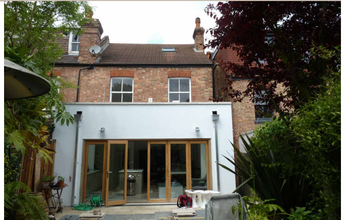
Case study: Loft conversion and dormer extension in Dulwich
